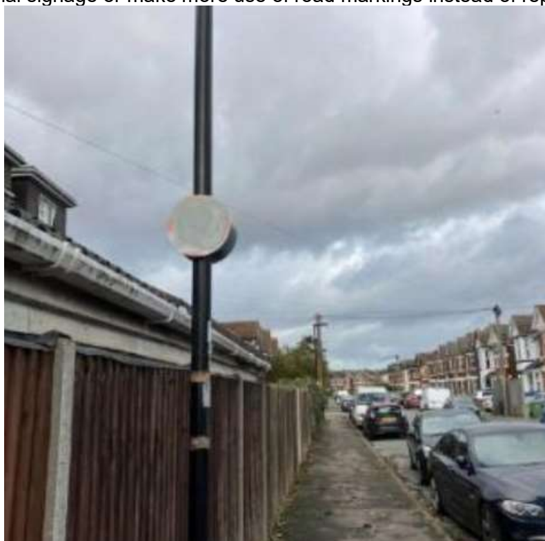
Figure 6 – Vandalised 20mph Repeater Sign
