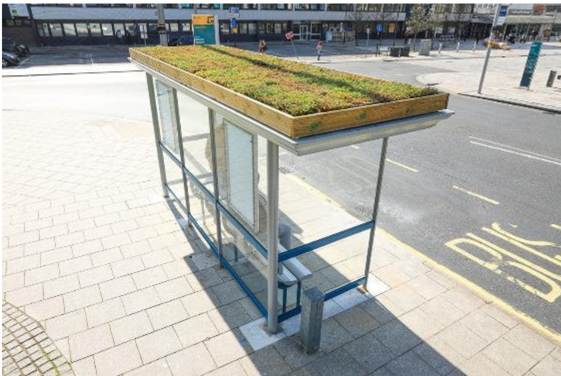
Figure 3.13 – Green roof bus stop at Southampton Central Station
